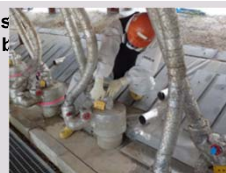
Commencement of Phase 2 freezing
