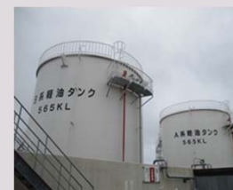
Light oil tanks for Unit 7 after replacement (Thickness of the steel plating of the tanks is approximately four times what it was)
