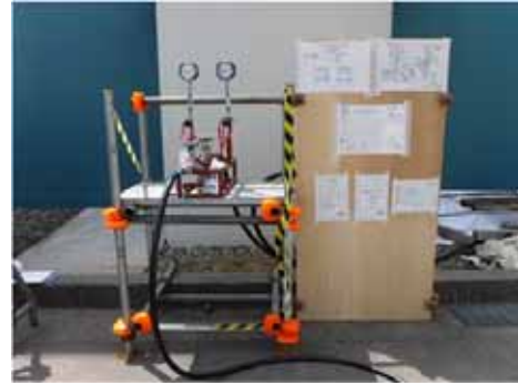
Pressure testing of pipes (Unit 6)
