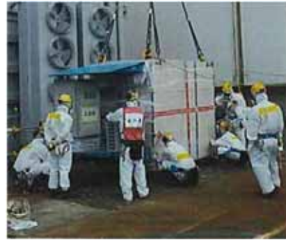
Installation of measurement device
