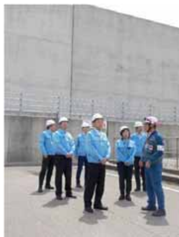
Tour of Kashiwazaki-Kariwa NPS (seawall)
