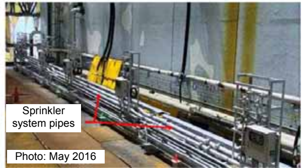
Installation of sprinkler system pipes
