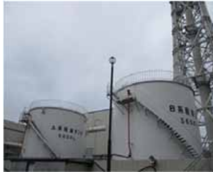
Light oil tanks at Unit 6
