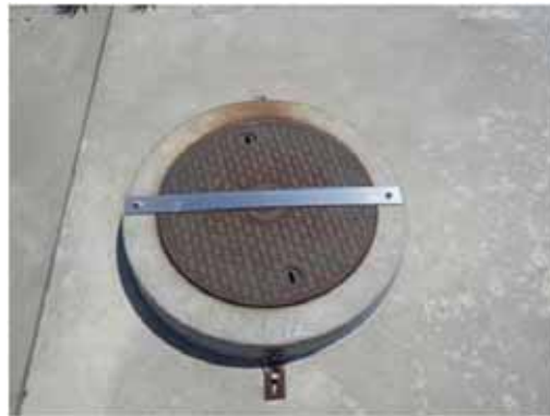
Anchored manhole cover
