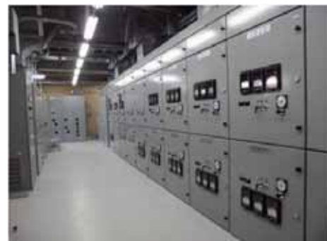
Emergency switchboard on the Arahama side
