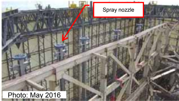
Installation of sprinkler system nozzle units
