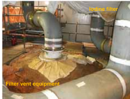
Pipes around iodine filter (Unit 6)
