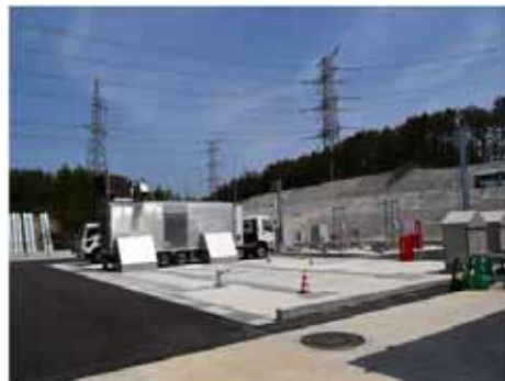
Additional air-cooled gas turbine power supply car
