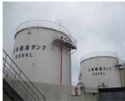
Light oil tanks at Unit 7
