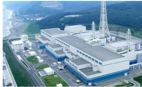
Kashiwazaki-Kariwa Nuclear Power Station
