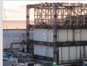
Wall panel removal completed
