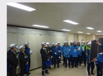
Unit 5 TSC construction area (Field inspection by the Nuclear Regulation Authority)
