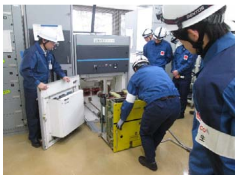
Training on handling high voltage and special high voltage electrical equipment
