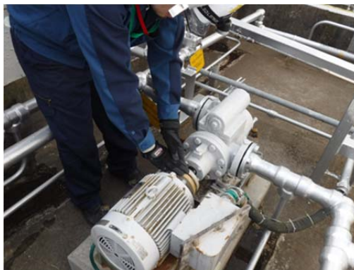
Manually operating fuel transfer pump
