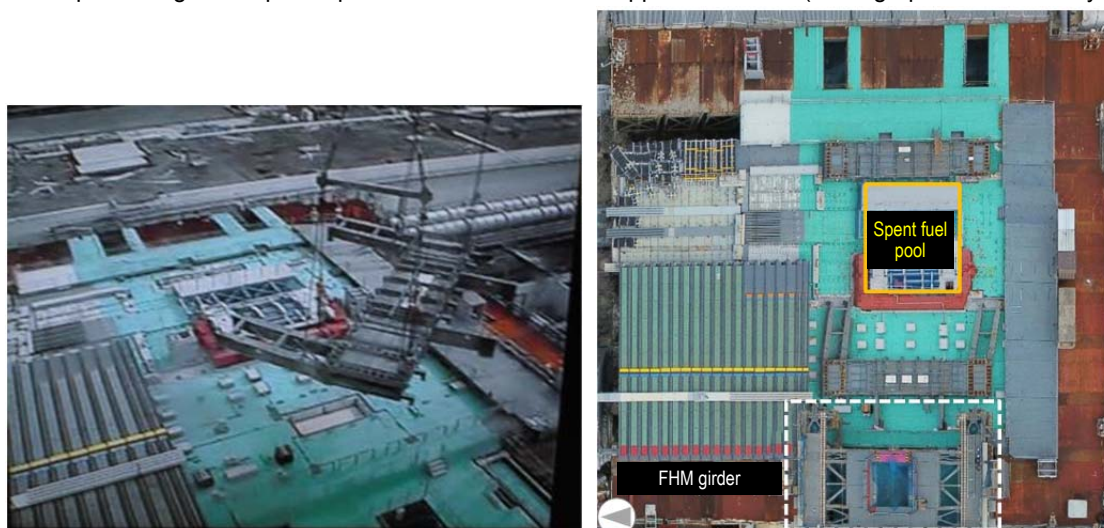
Stopper installation (Photographed on February 7) FHM girder construction (Photographed on March 13)
