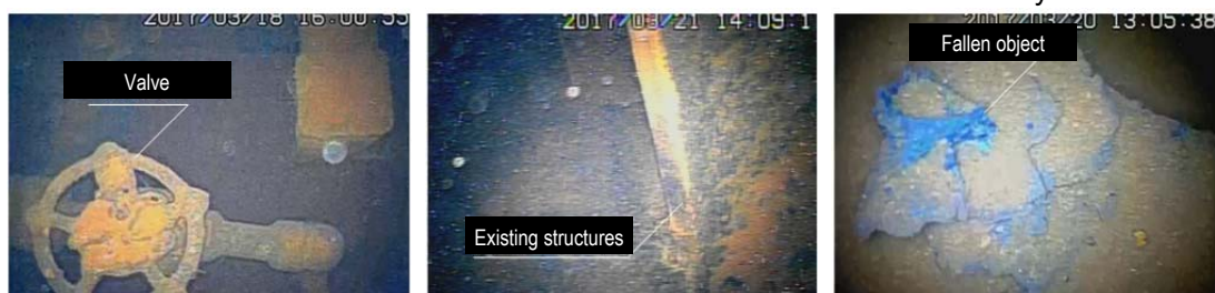
Photographs from Unit 1 PCV internal survey
