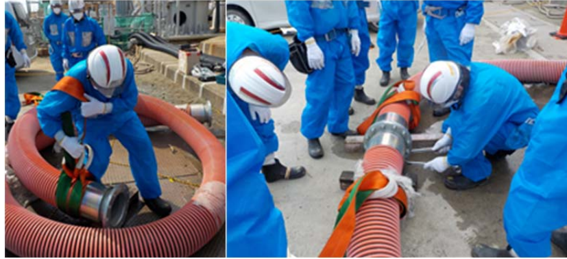
Training on laying and connecting temporary hoses (Left: Moving and laying hoses, Right: Connecting flanges)
