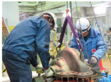
Horizontal pump disassembly inspection training (casing lowering)
