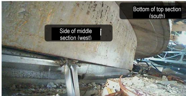
Damage to reactor well plug
