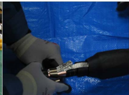
High voltage cable splicing training (Left: Cable cutting/shield removal, Left: Splicing)
