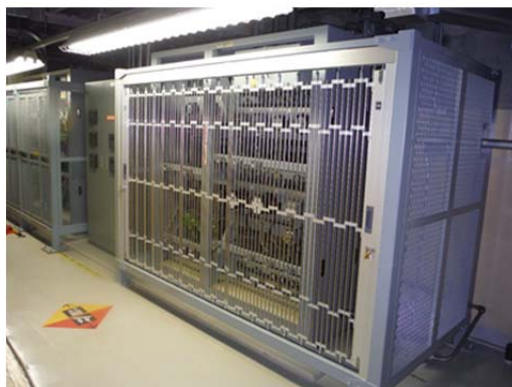
Installation of protective fence around instrument rack
