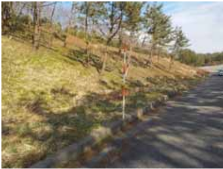
Prior to asphalt paving
