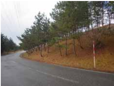
Prior to fire belt creation
