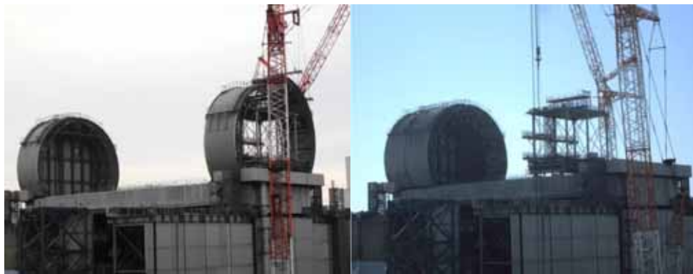
Dome roof installation (Left: September 6, Right: September 26)
