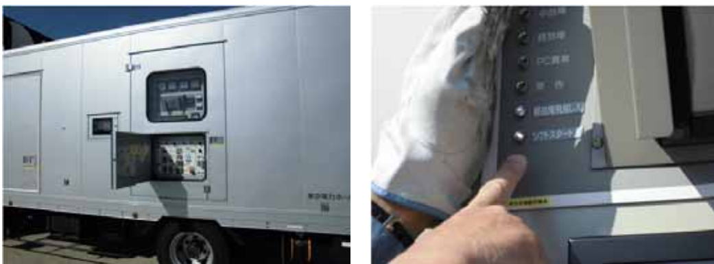
Generator truck improvements (left: Exterior view, right: Control panel)
