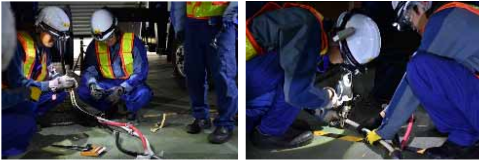
Temporary cable connection training simulating nighttime conditions
