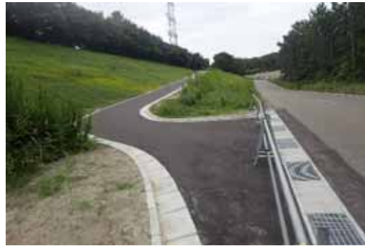
After asphalt paving
