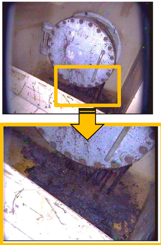
Figure 3-13 Melted matter at the penetration flange [27]
