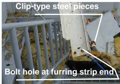
(B) Bolt hole at furring strip end
