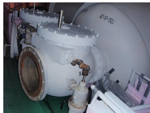
Figure 2 Vacuum breaker valve
