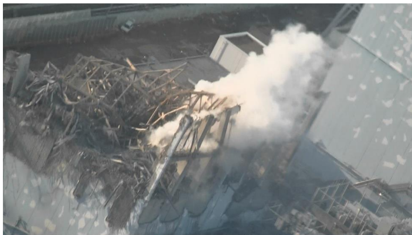
Figure 12 Aerial photo of Unit-3 (March 16 th , 2011)
