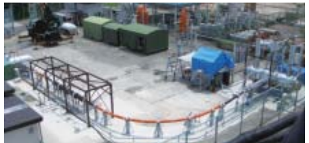
External view of a 30-meter HTS cable test system at Sumitomo Electric Industries, Ltd.'s Kumatori Works Joint development with Sumitomo Electric Industries
