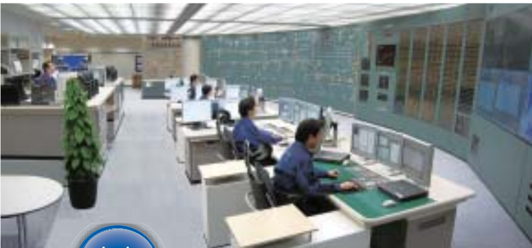
Central load-dispatching office
