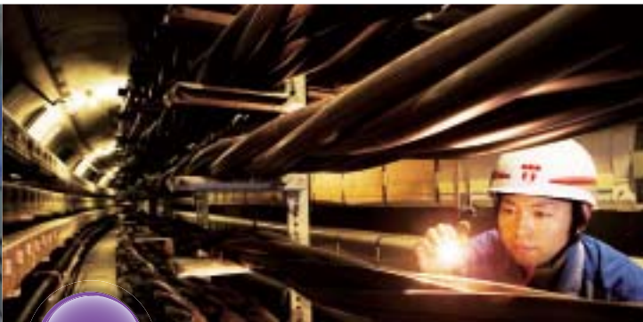
Inspection of underground power transmission
