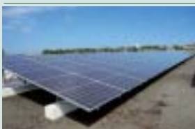
Ohgishima Solar Power Station (under construction)
