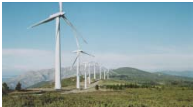
Paxareiras, Spain, Eurus Energy Holdings Corporation
