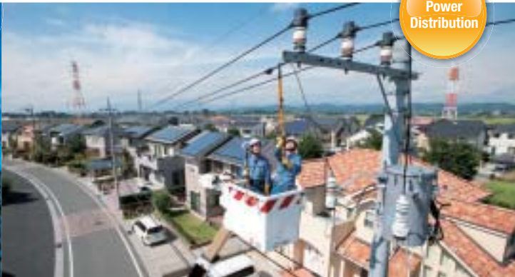
Inspection of high-voltage power distribution lines (indirect work)
