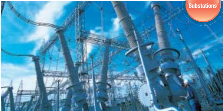
New Fukushima Substation
