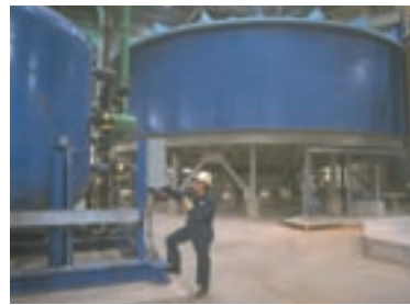
Inside of the McLean Lake Mill, Canada
