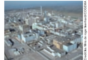
COGEMA's UP-3 Reprocessing Facility (La Hague, France)
