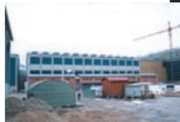
Interim storage facility Wuerenlingen (Switzerland)
