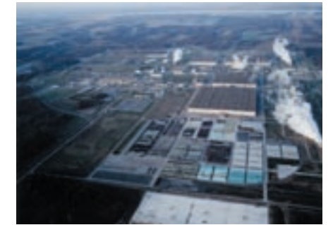
USEC's Paducah Enrichment Plant (U.S.)
