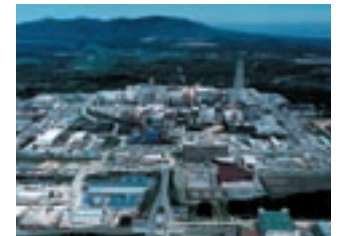
JNFL's Rokkasho Reprocessing Facility (under construction, Rokkashomura, Aomori Pref.)
