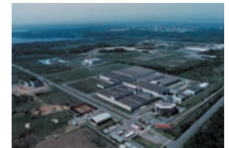
JNFL's Uranium Enrichment Plant in Rokkashomura, Aomori Pref. (Japan)
