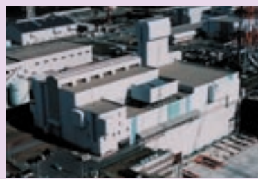
JNFL's Vitrified Waste Storage Center (Rokkashomura, Aomori Pref.)
