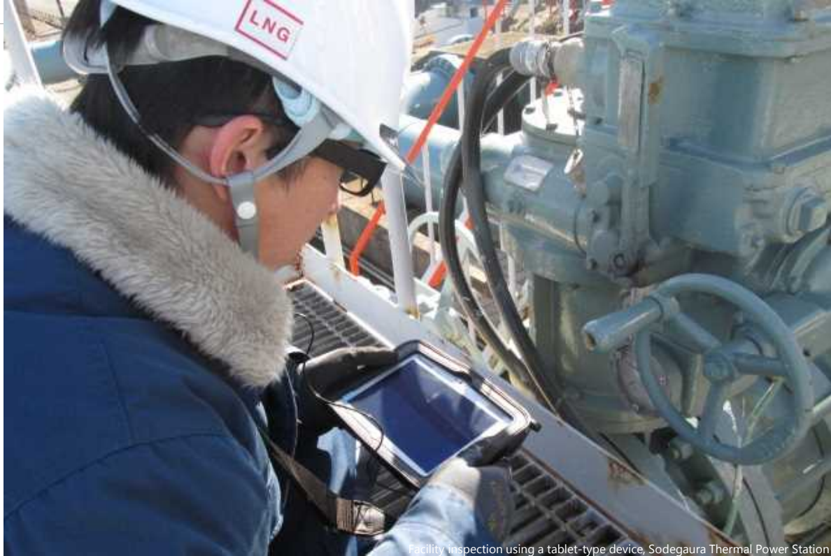
Facility inspection using a tablet-type device, Sodegaura Thermal Power Station
