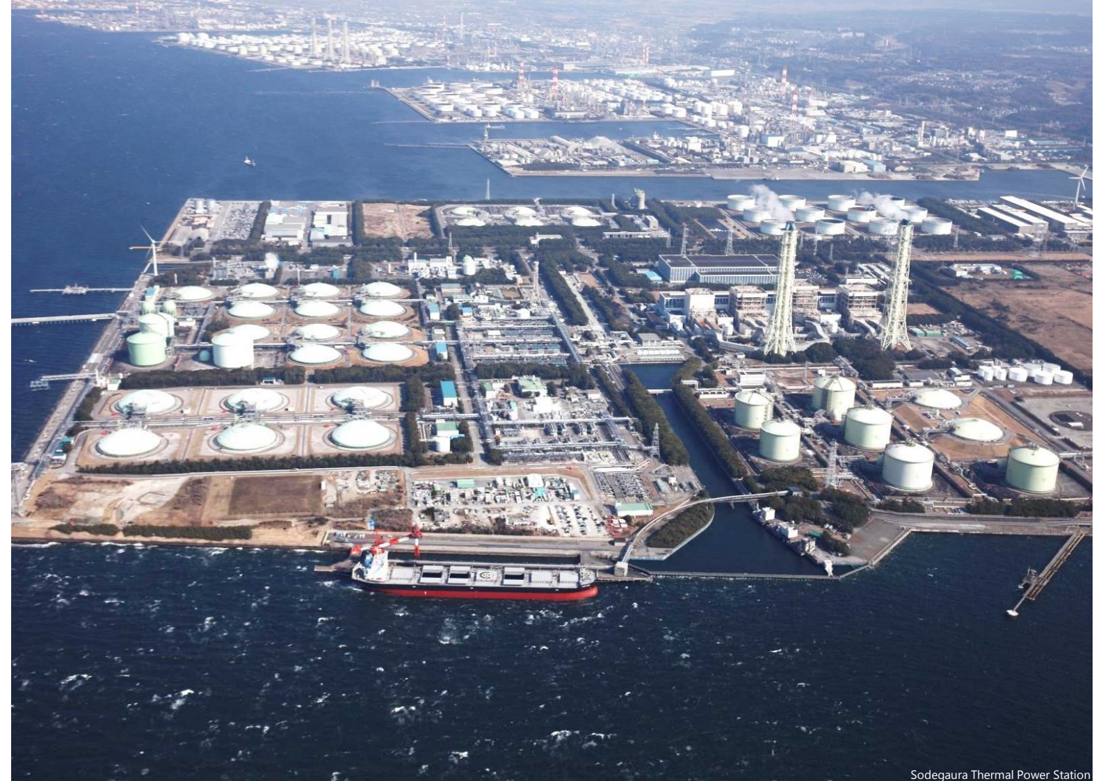
Sodegaura Thermal Power Station
