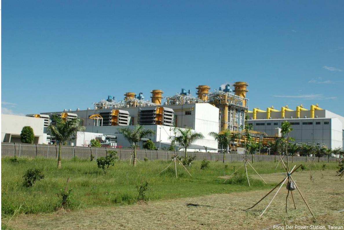
Fong Der Power Station, Taiwan
