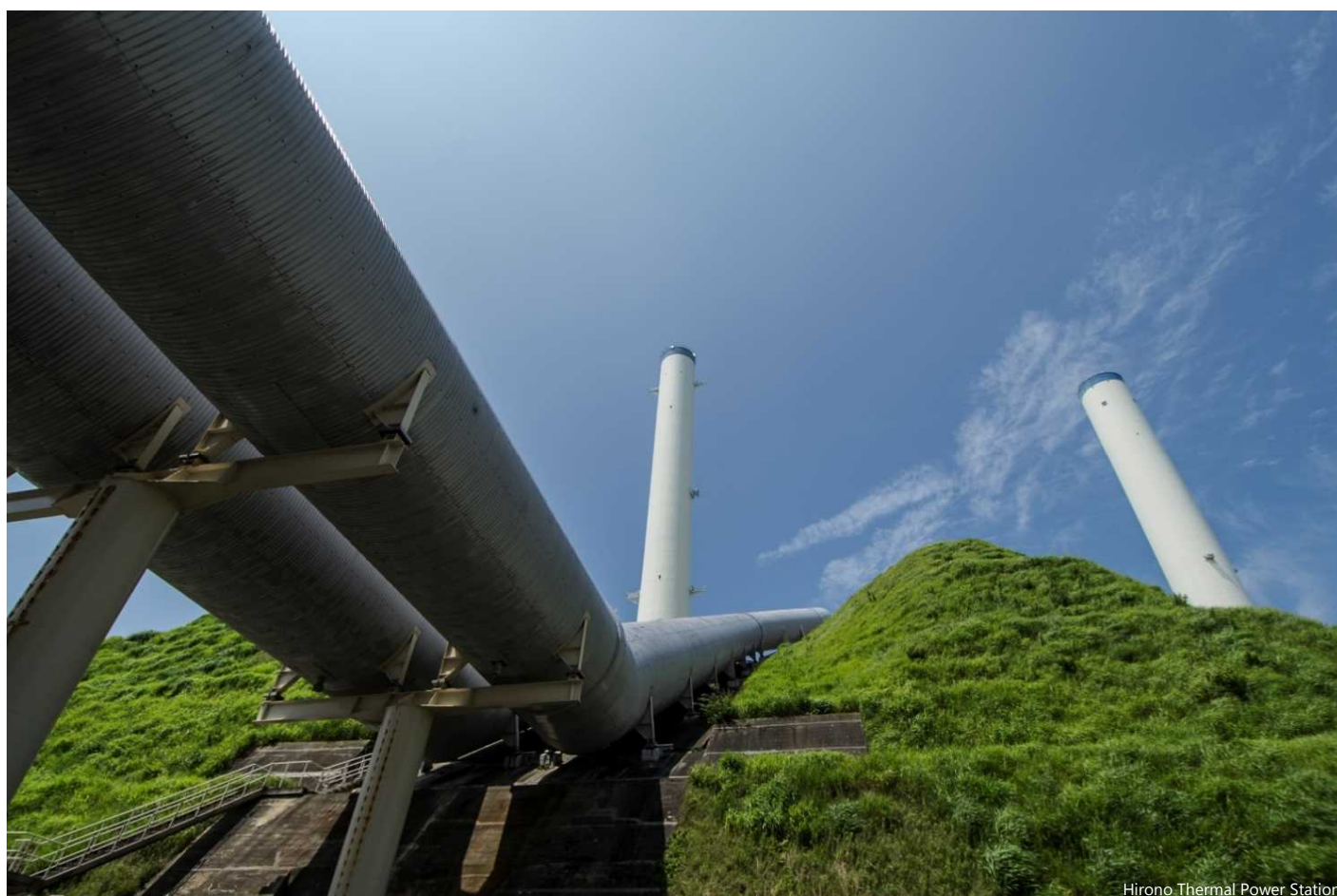
Hirono Thermal Power Station
