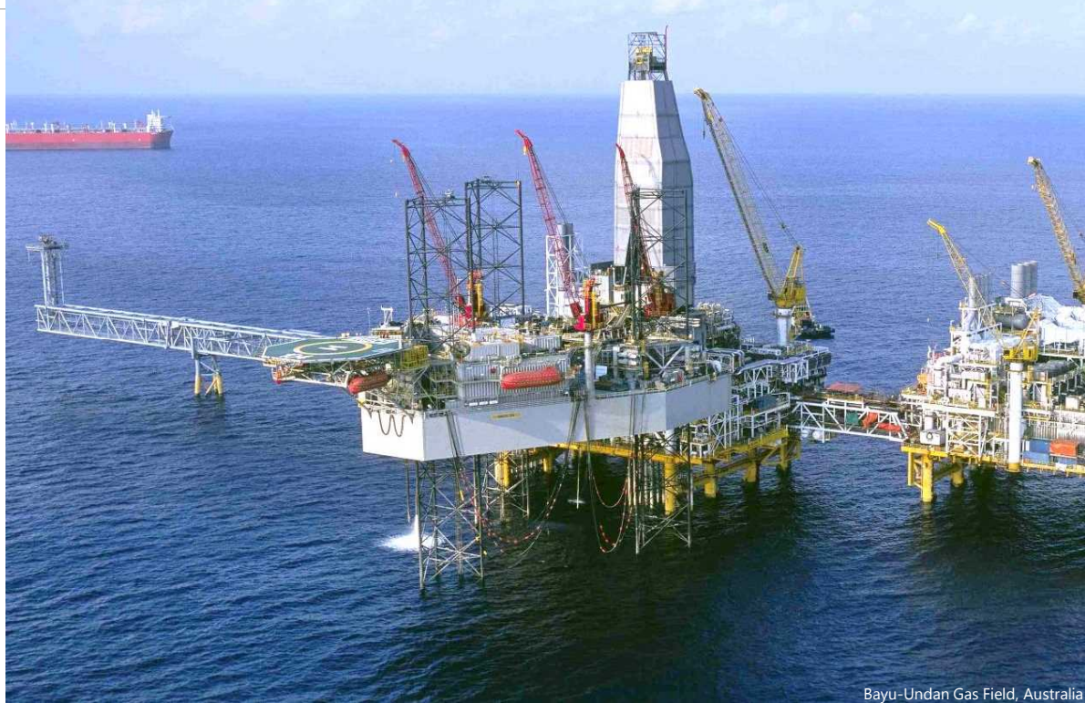
Bayu-Undan Gas Field, Australia
