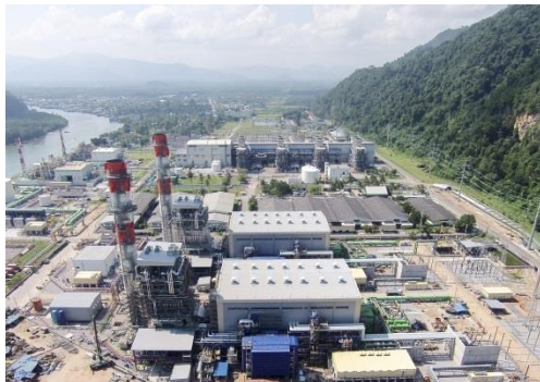
Khanom Power Station, Thailand
