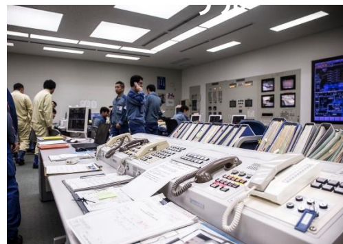
Central operation room of Kawasaki Thermal Power Station
