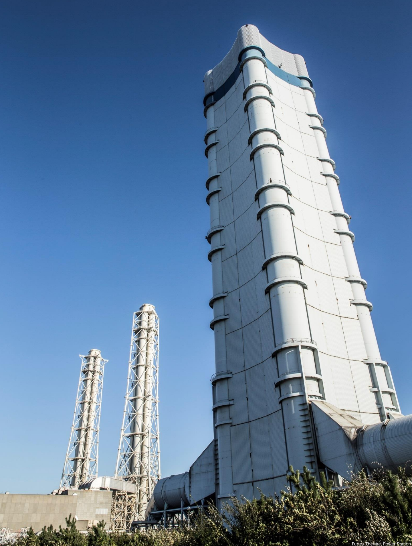
Futtsu Thermal Power Station
