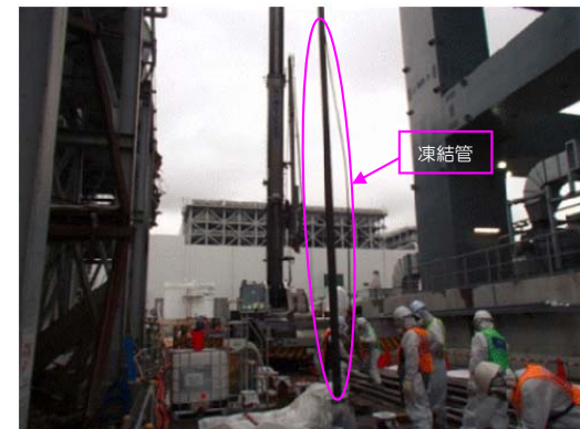
<凍結管設置の状況>
