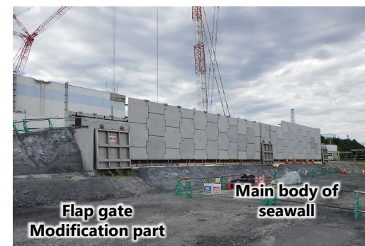
[Picture ②] North side seawall under construction (2022.8)
