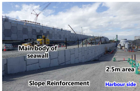
[Picture ①] Main body of seawall under construction (2022.9)
