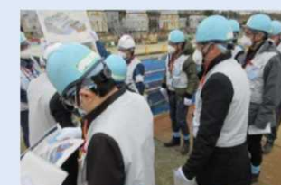
Inspection around the discharge vertical shaft
