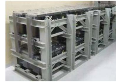
DC Power Supply Equipment (Equipped at Elevation in the Reactor Buildings)
