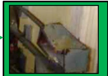
Distorted pull box (downward distortion)
