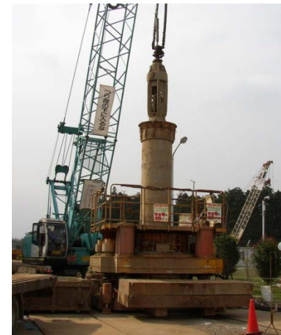
An image of soil improvement
