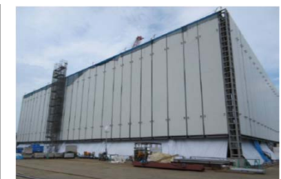
Exterior of the bldg. of Improved ALPS
