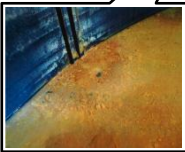
Prior to sludge removal
