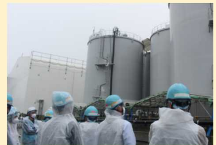
K4 tank area
