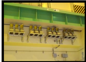
Passive autocatalytic recombiner (PAR)
