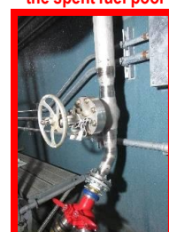
External connecting port to inject water into the spent fuel pool
