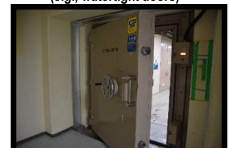
Inundation protection measures (e.g., watertight doors)
