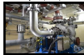
High-pressure alternate cooling system (HPAC)
