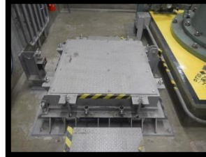
Intake tank stoppage plate
