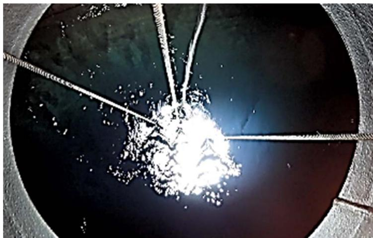
Water surface in the tank while the Agitation equipment is in operation (Picture shot at T/R)
