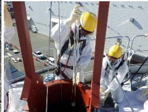
Water sampling on the day of the agitation demonstration test
