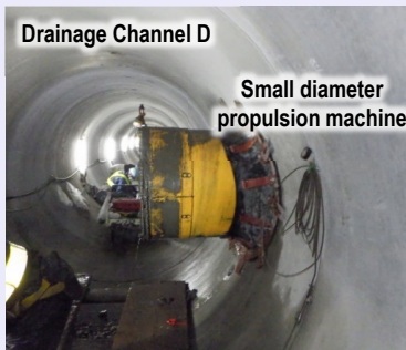
<Construction status of Drainage Channel D> (Small diameter propulsion work)
