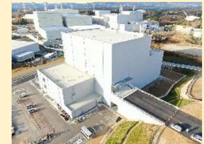
Whole view of the Additional Solid Waste Incinerator Building
