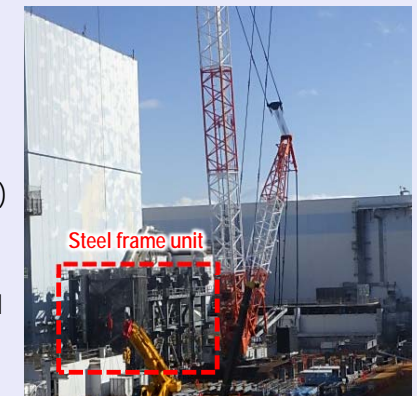
< Whole view of Unit 2 Reactor Building south yard (February 10, 2023) >
