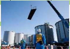
Construction of welded-joint tanks
