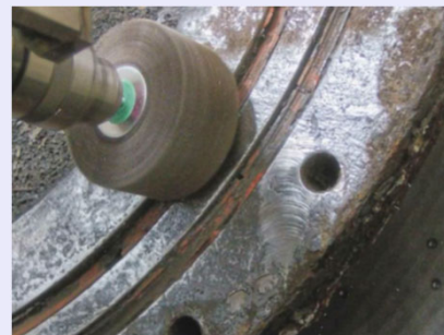
< Cleaning of X-6 penetration flange surface >
