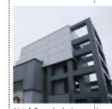
<Unit 4 Cover for fuel removal>
