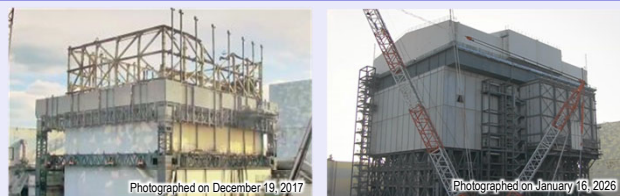
Unit 1 Reactor Building prior to cover installation
