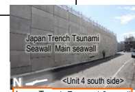
Japan Trench Tsunami Seawall
