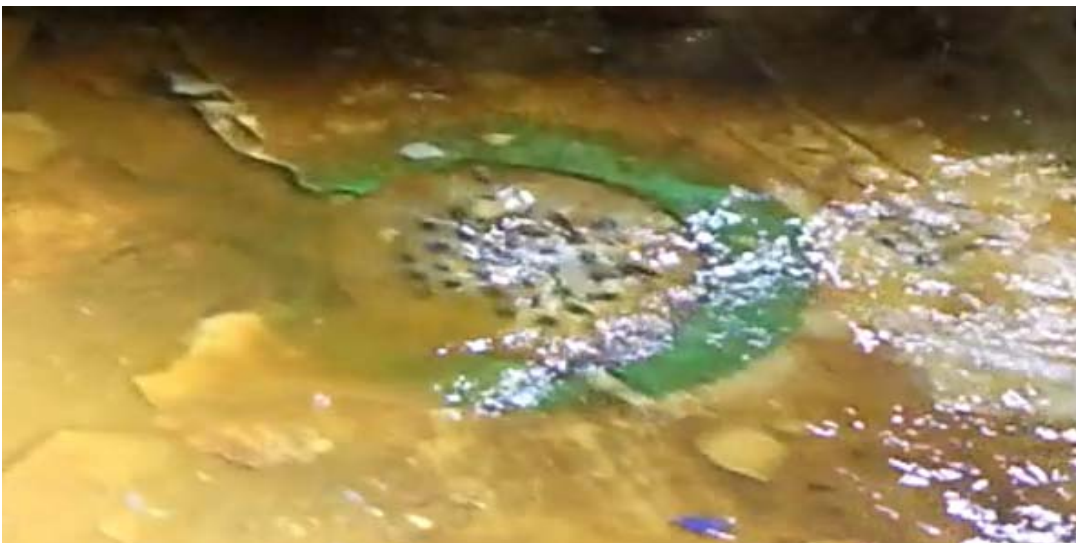
Water flowing again through cleaned funnels (Water is flowing into the southeast triangular corner of the subfloor)
