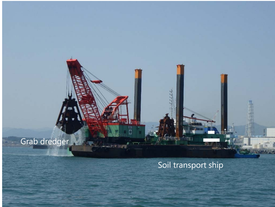
Offshore excavation
