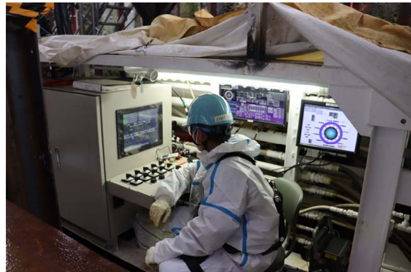
Status of shield machine drilling ②
