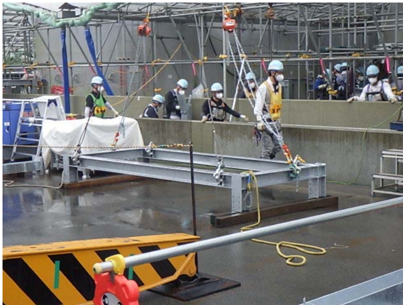
Status of circulation pipe support installation
