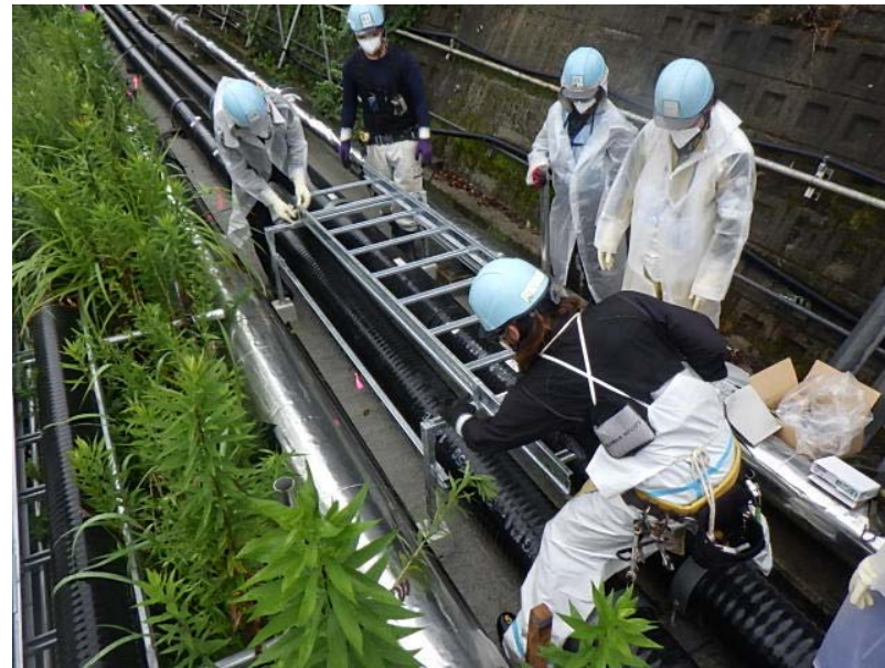
Status of transfer pipe support installation
