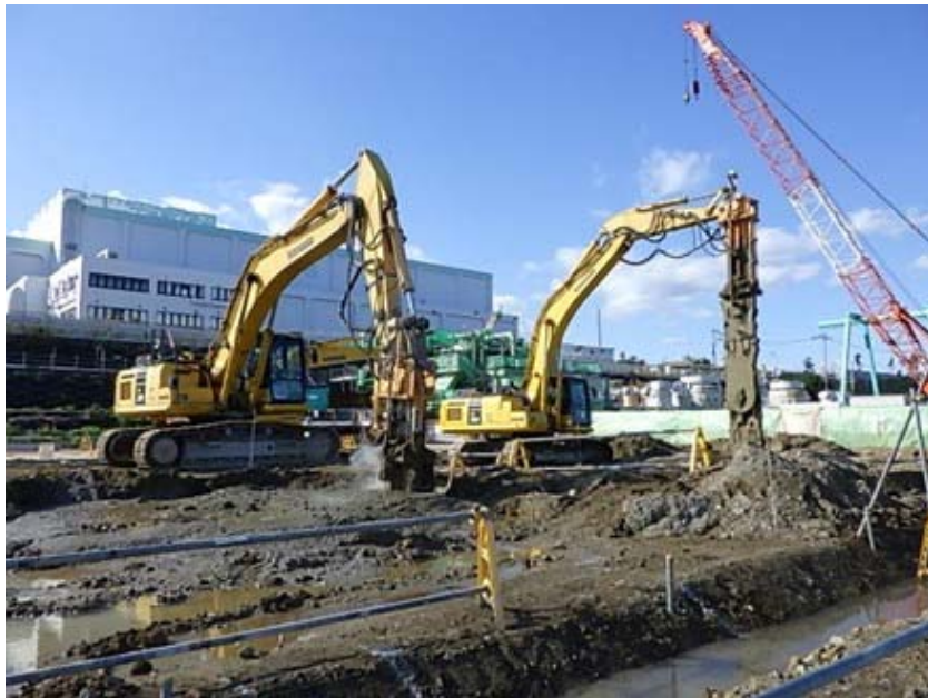
Ground improvement work
