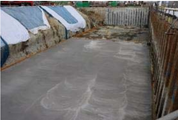
Placing leveling concrete
