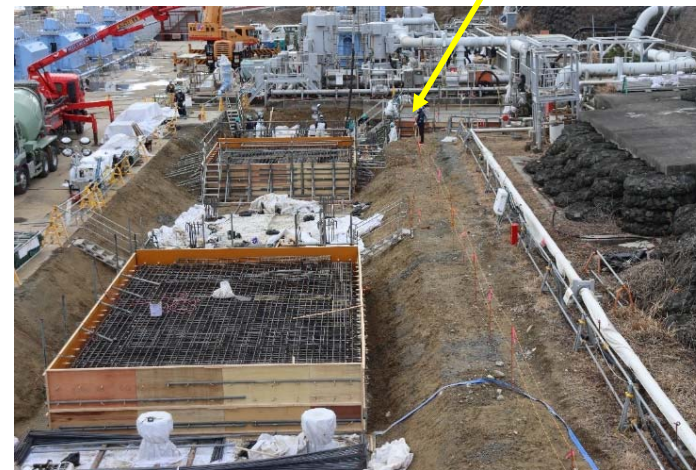
Building the seawater transfer pipe foundation
