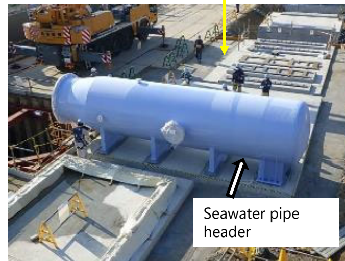
Building the seawater transfer pipes foundation and installing the seawater pipe header
