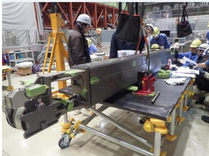
Arm maintenance/internal cable replacement
