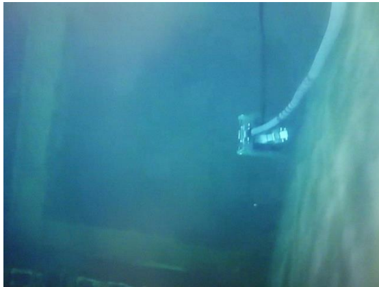
October 21, 2025 Deploying the submersible cleaning robot into the cask pit
