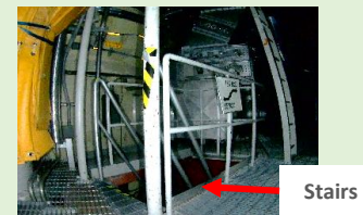
③ Subfloor stairs (south)
