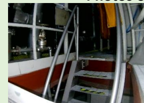
① Subfloor stairs (north)
