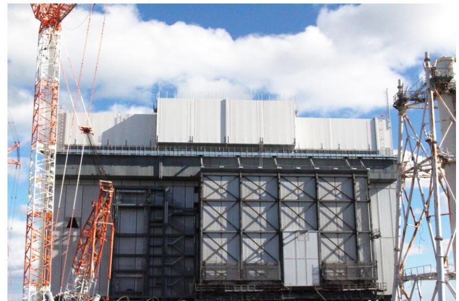
A retractable roof has been installed. The photo shows the roof when completely close (Photographed from the west) (Photographed on January 16, 2026)
