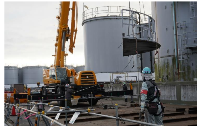
< The top Lid removed from J8 area tank >
