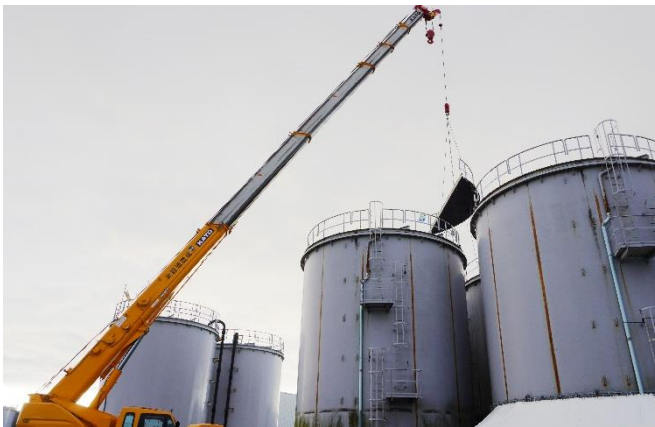
< Removing the top lid from J8 area tank >
