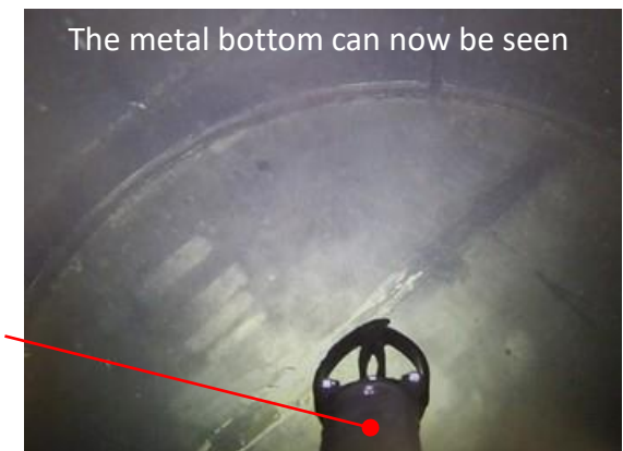
Bottom of cask pit after cleaning (Photographed on November 5, 2025)
