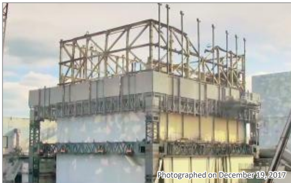
Unit 1 reactor building prior to cover installation
