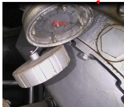
3A valve opening angle gauge (indicates full open)
