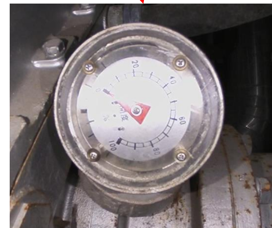
3B valve opening angle gauge (indicates full open)
