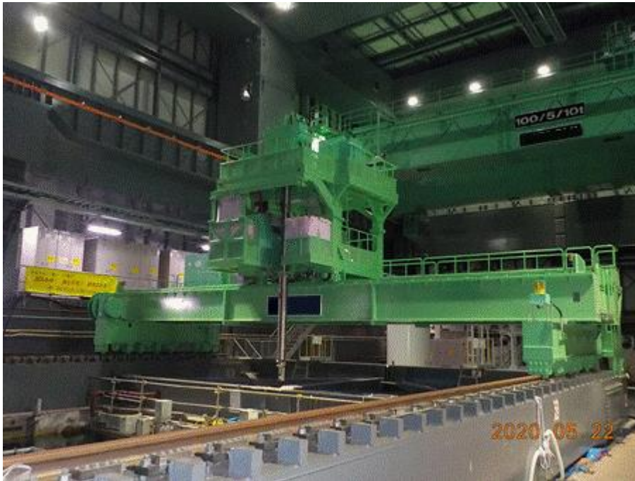
Prior to removal of the fuel handling machine (Photographed on May 22, 2020)
