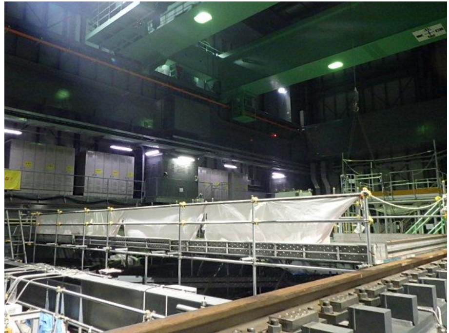
After removal of the fuel handling machine (Photographed on February 18, 2026)
