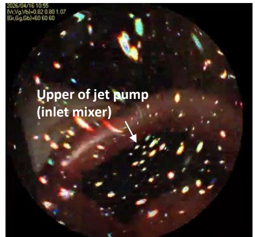
Photo ③ Approx. 1m below N16A nozzle
