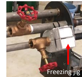
Refrigerant (dry ice + alcohol) replace regularly
