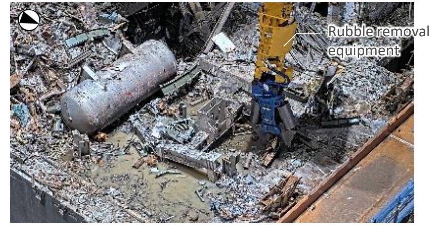
Relocating rubble (photographed on May 21, 2026)
