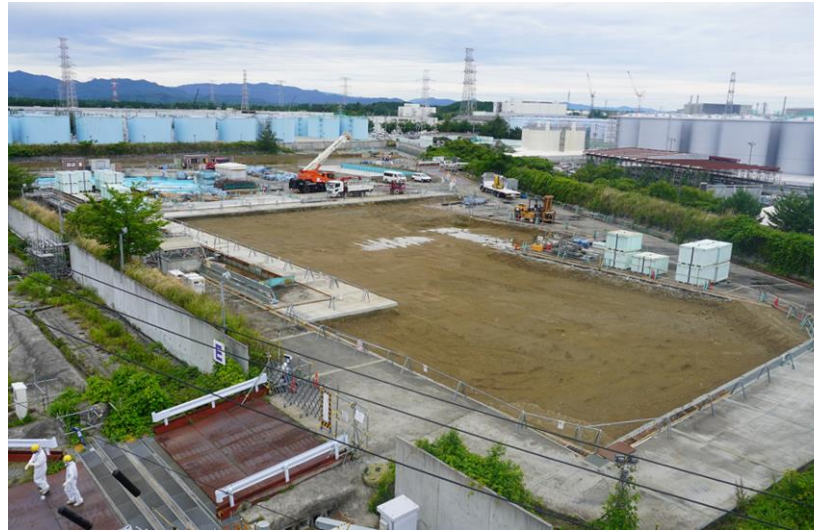
After dismantling D1 tank in E area (June 15, 2026)
