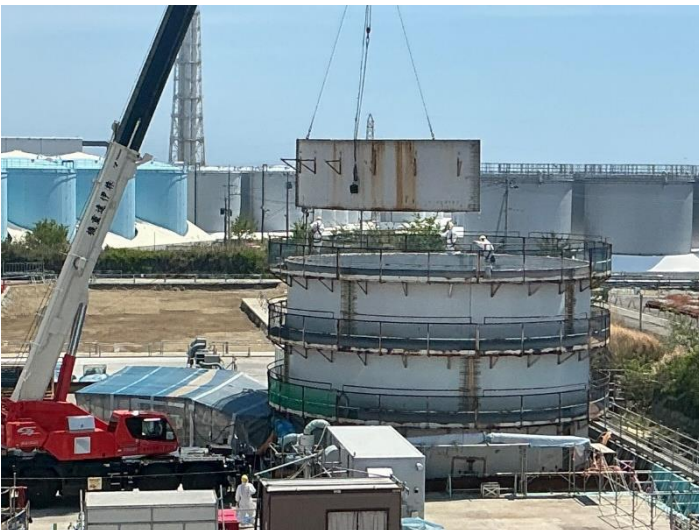
Dismantling of D1 tank in E area (May 12, 2026)
